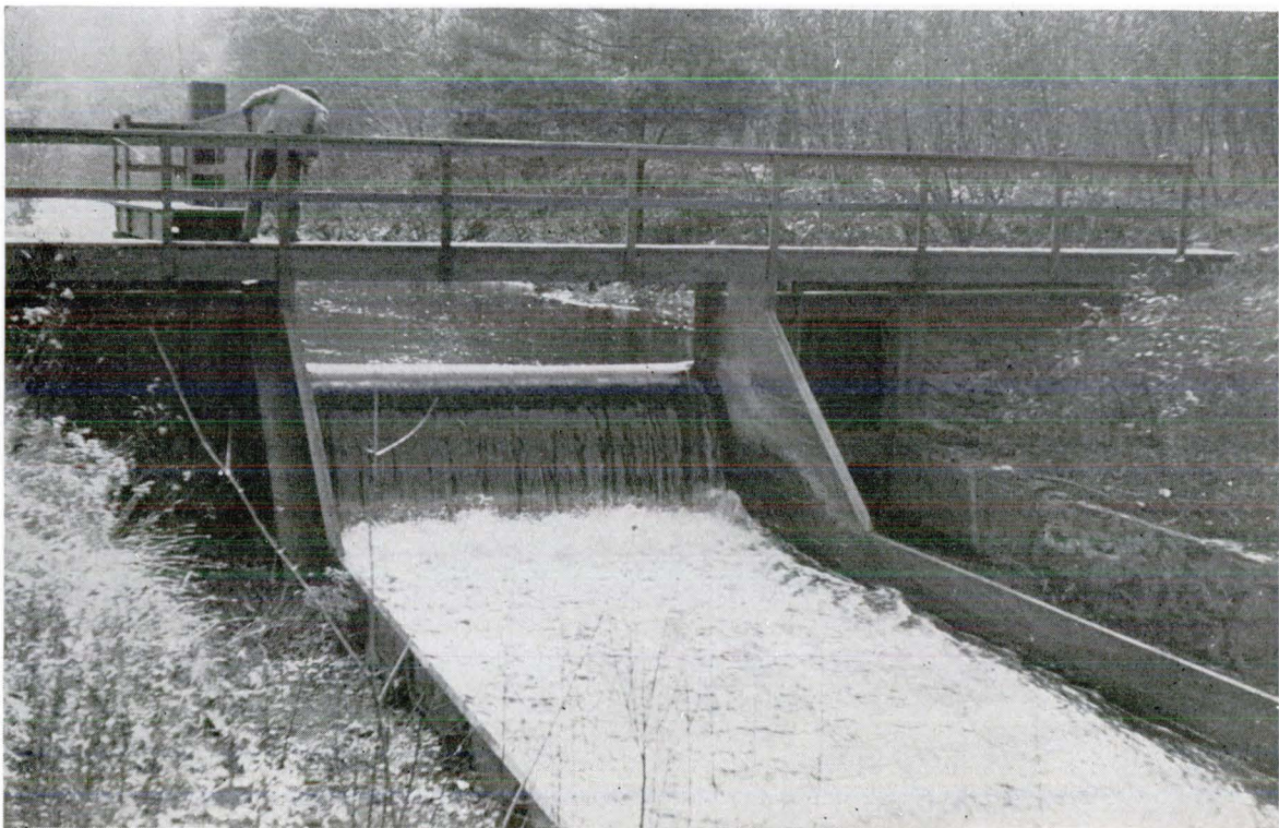
FIGURE 13.—Weir installation for measuring mine-water drainage.
