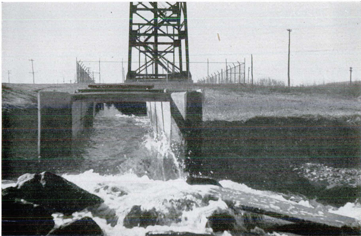
FIGURE 9.—Mine pump discharging 260,000,000 gallons a month into a breaker storage pond.
