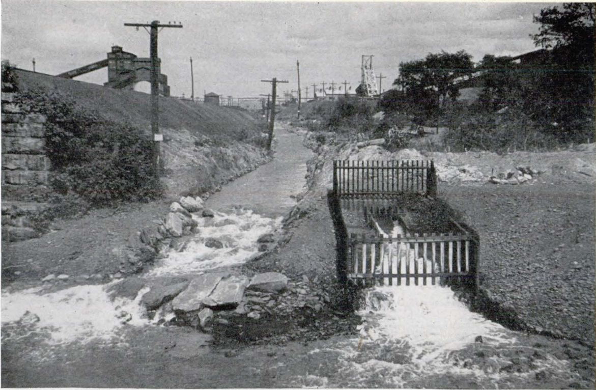
FIGURE 10.—Two discharges, totaling 24,000 g. p. m., from one colliery in the Northern field.
